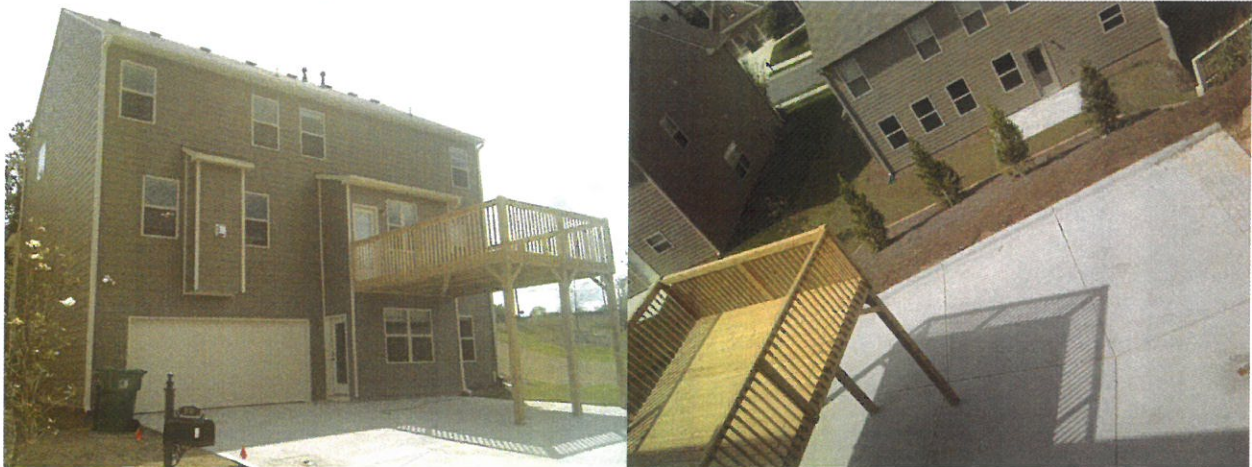
Deck when Home was Purchased:
