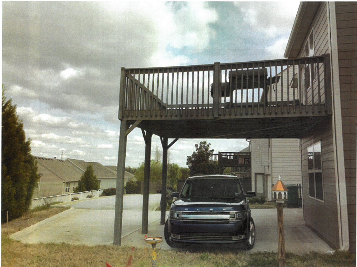
Deck at Present:
