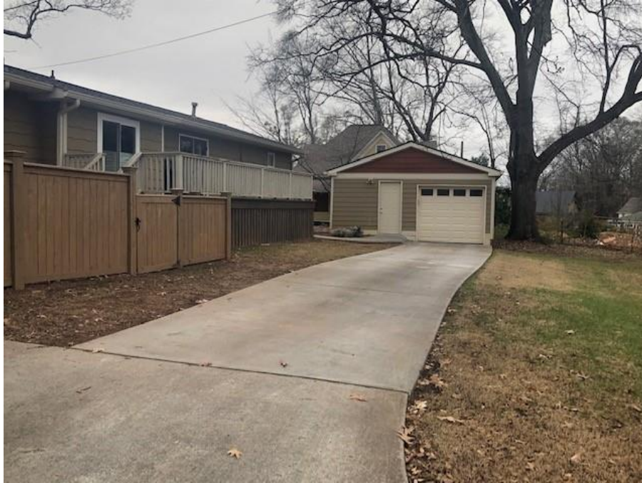
Figure – 4 Existing Detached Garage and Driveway to be Removed
