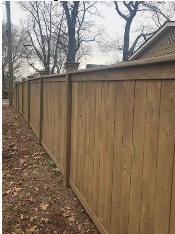
Figure – 4 Existing 5.6-foot Wooden Fence
