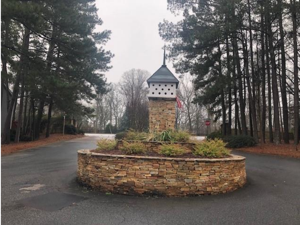
Figure – 7 View to the South
