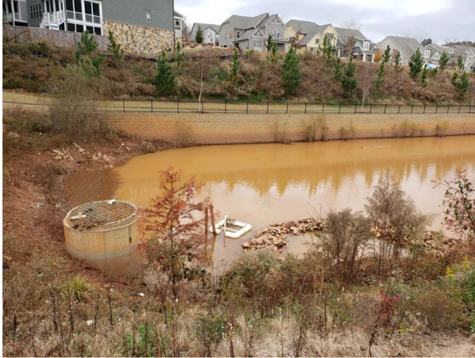
3. View of retention pond (lake).
