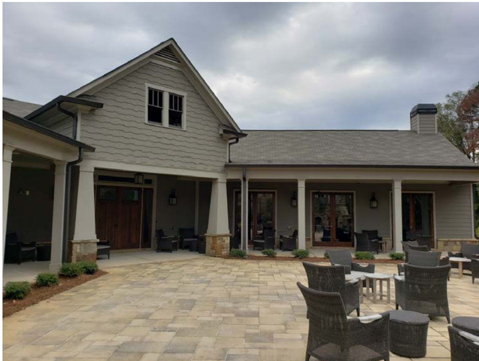
10. View of rear elevation of the clubhouse.
