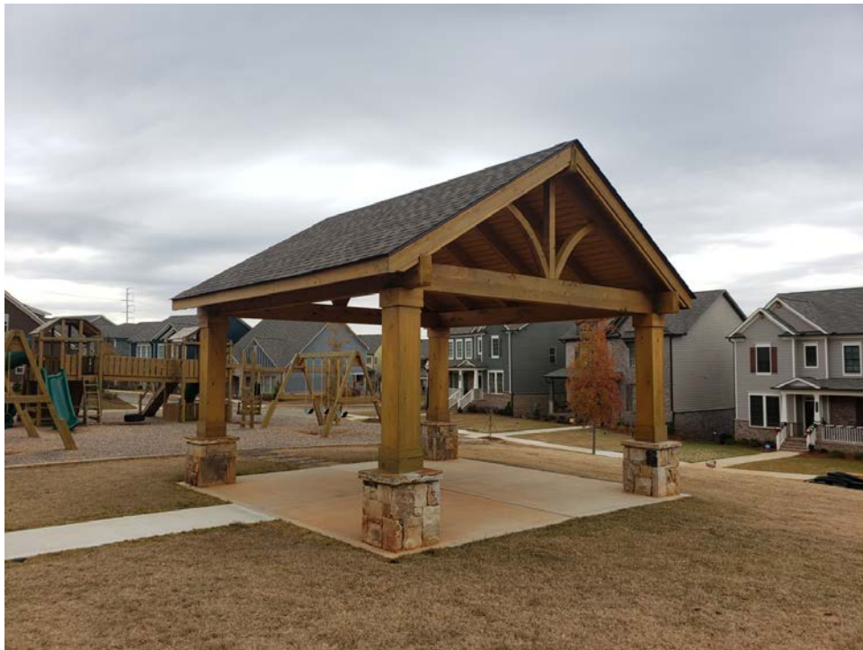
14. View of pavilion.
