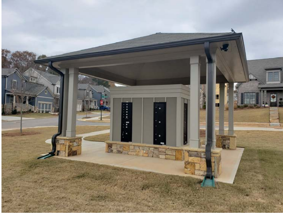
15. View of mailbox kiosk.
