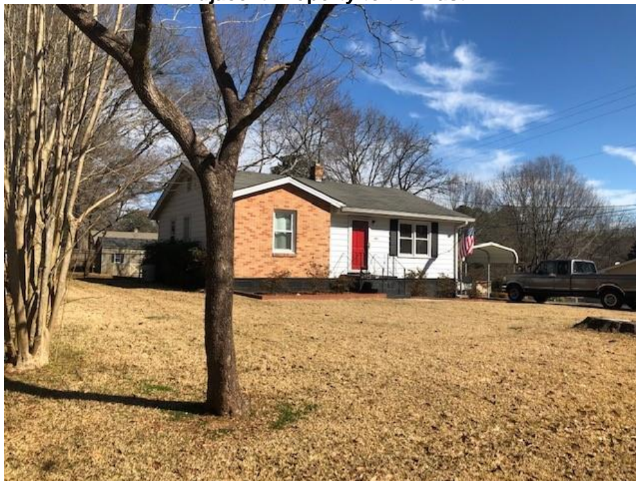
Figure – 6 Adjacent Property to the East
