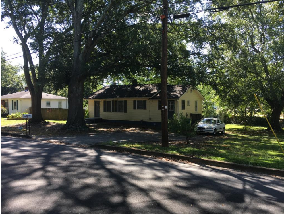
Figure – 2 (Adjacent Properties)
