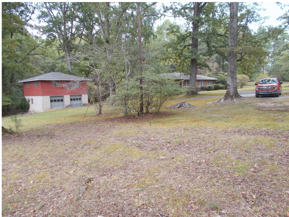
Transect 1, Shovel Test 1, Middle 20 th Century Structure Complex, Facing North-Northeast
