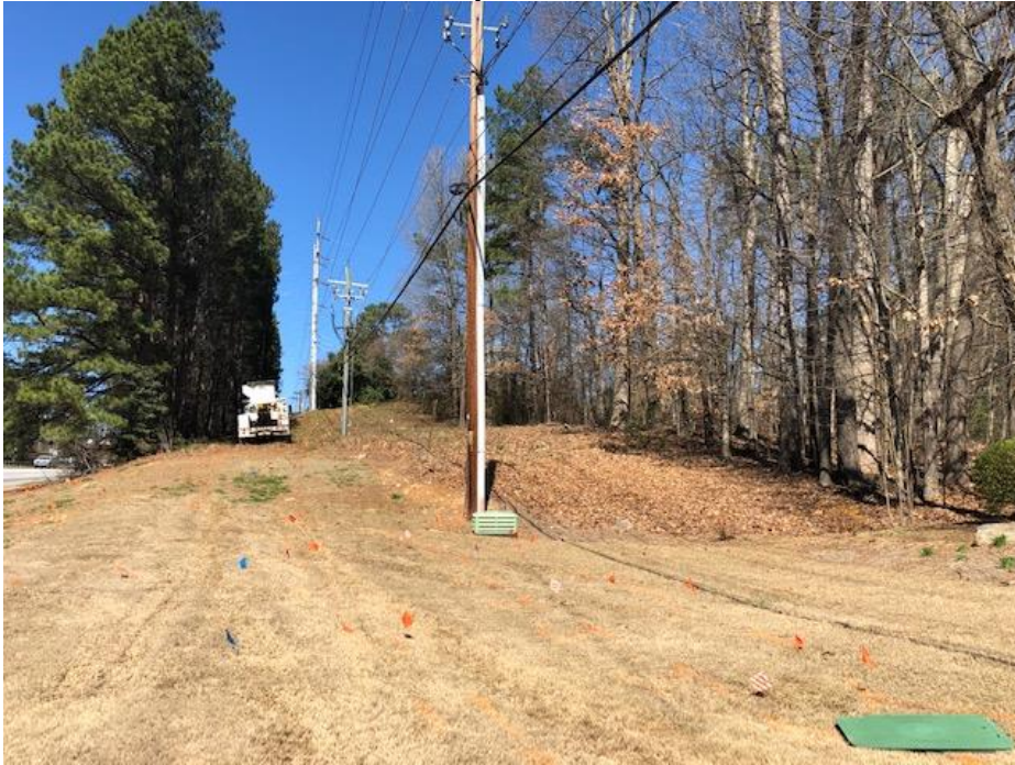
Looking north along S. Cobb Drive towards power station
