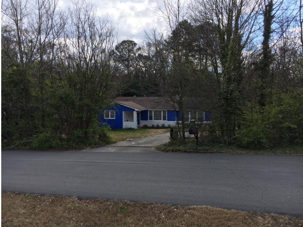
Figure – 2 Adjacent Properties
