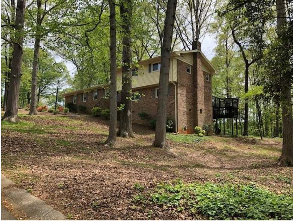
Figure – 8 Adjacent Property to the East
