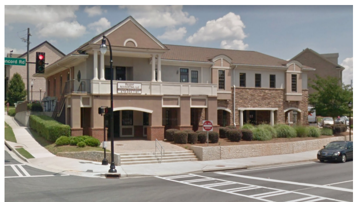
Office building on Concord Road
