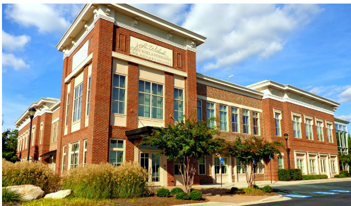
Office building on Atlanta Road
