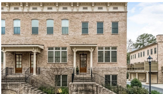
Townhomes in the Ansley Park neighborhood of Atlanta
