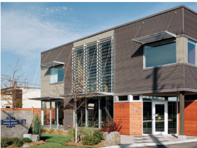
Sustainably designed light manufacturing facility
