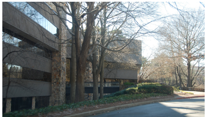
Office park campus on S. Cobb Parkway
