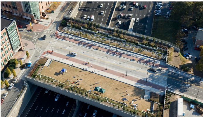
Fifth Street bridge at Georgia Tech, designed to enhance connectivity and minimize highway impact on the pedestrian experience
