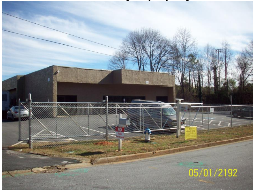
Figure – 2 View of subject property
