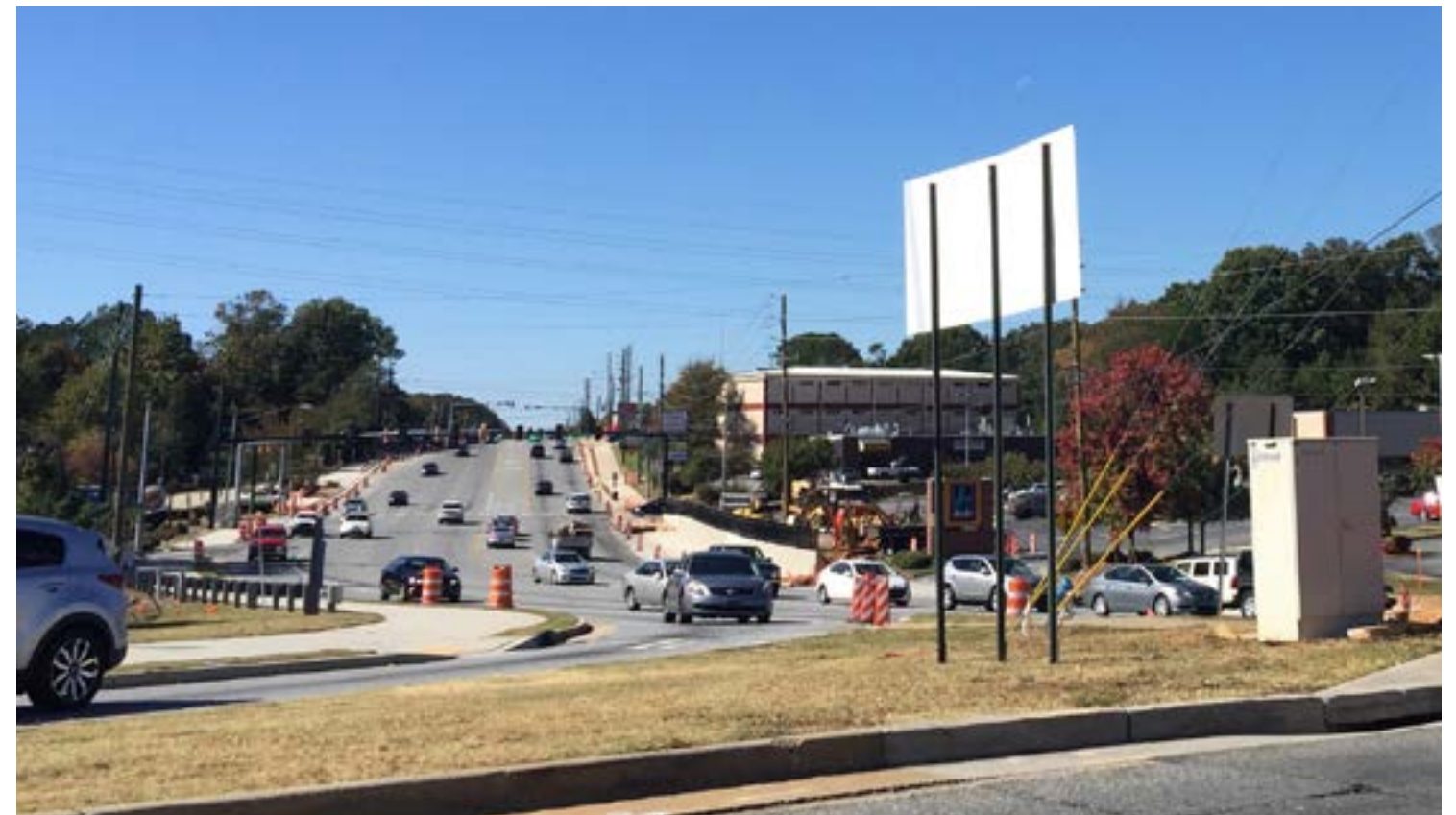
FIGURE 10 LOOKING WEST ON SPRING ROAD. IMPROVEMENTS UNDERWAY INCLUDE ROADWAY WIDENING NEAR THE CUMBERLAND BLVD. AND COBB PARKWAY INTERSECTIONS, AS WELL AS THE ADDITION OF MULTI-USE TRAILS ON BOTH THE NORTH AND SOUTH SIDE OF THE CORRIDOR.
